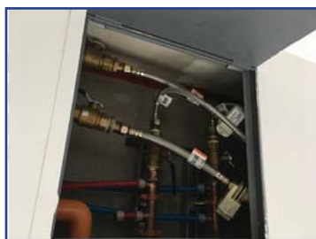
Figure 3. Two water meters are configured for point-of-entry monitoring for each unit at 360 State Street.
